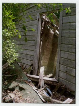
(a) Front of residence structure; collapsed front porch under composite roof panel, facing southeast.
