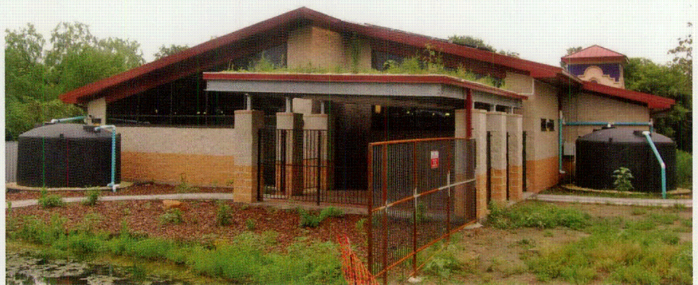
Retrofitted Valley Nature Center (Source: Texas A&M University-Kingsville)
