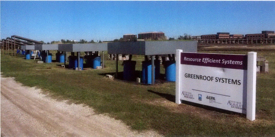
Green roofs and collection systems (Source: Texas A&M AgriLife Research)
