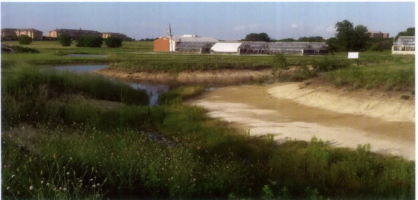
Meandering detention pond (Source: Texas A&M AgriLife Research)
