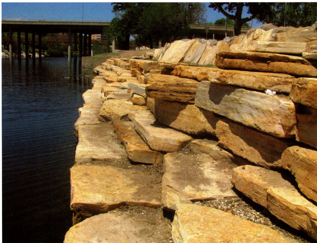
North Concho River with bank stabilizing BMPs
