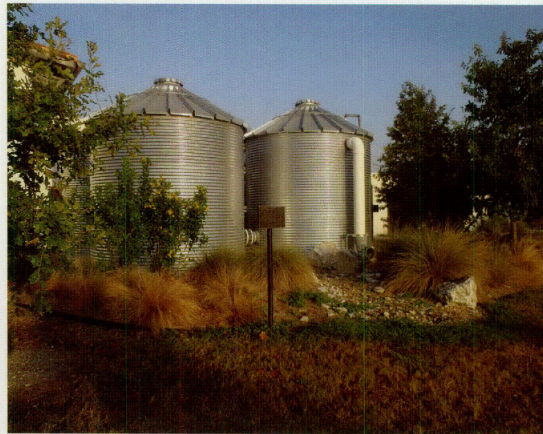
Cisterns in rain garden at redeveloped Mission Drive-In Theater (Source: San Antonio River Authority)
