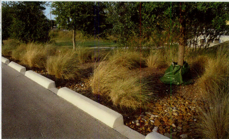
Parking lot bioswale at the redeveloped Mission Drive-In Theater (Source: San Antonio River Authority)
