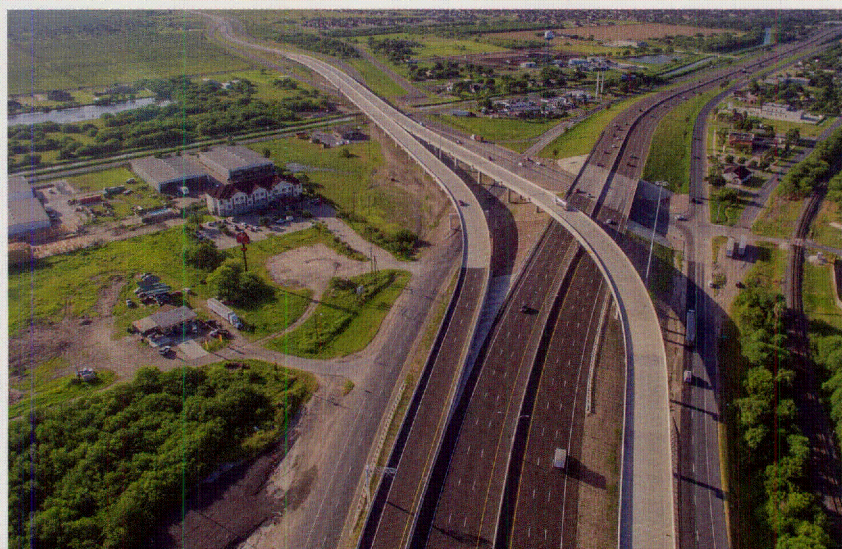
SH 550 opened for traffic near Brownsville in June. The toll road provides a faster route for truck traffic to the Port of Brownsville. Photo courtesy of the Cameron County Regional Mobility Authority.
