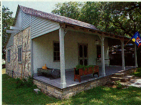
Founded by German freethinkers in 1854, the Central Texas town of Comfort carefully preserves its heritage. The 1860 Michael Lindner cabin (above) and the 1860 Otto Brinkmann Cottage (detail, below) display fachwerk , a style of construction that fills exposed, heavy-timbered framing with native stone.
