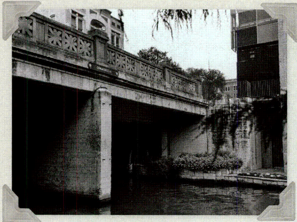
Commerce St. Bridge
