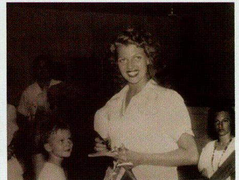
Built in 1903, the sprawling Luther Hotel (left) offers charming rooms, including Luther's Penthouse, the only room with a balcony. Rita Hayworth's picture adorns the Luther's walls, recalling her stay at the hotel while entertaining Camp Hulen troops during World War II.
