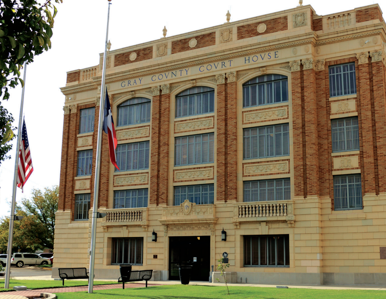
The Gray County Courthouse in Pampa was restored to its original Beaux Arts appearance thanks to the THC's courthouse preservation program.
