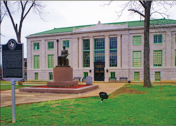
By participating in the Texas Courthouse Stewardship program, San Augustine County officials and employees can seek free professional advice from the THC's preservation architects.
