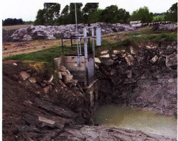
The images above show the outlet control structure from McLeod Hood Reservoir. The District replaced the gate and cut the concrete box down to allow for more flow from the reservoir.
