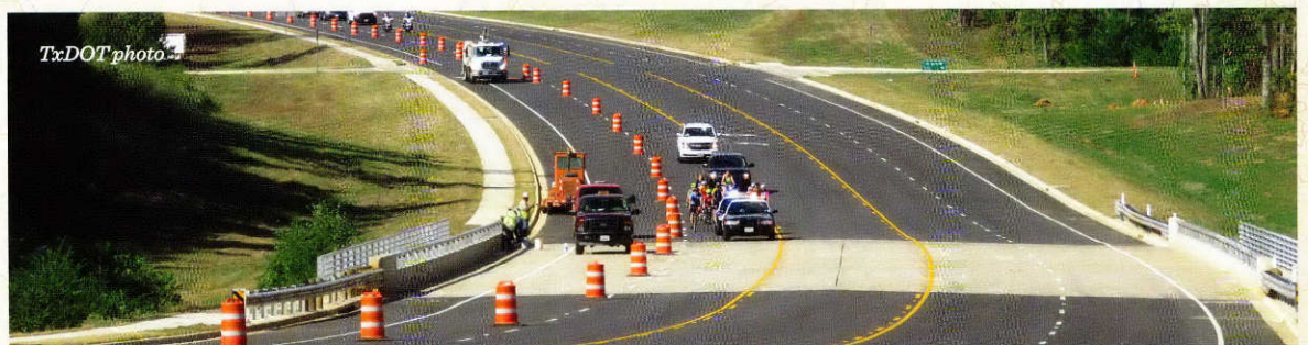
A portion of the FM 2275/George Richey Road Extension in the Tyler District opened to traffic in October. A biking tour on the new road was one of the highlights of the ribbon-cutting event.
