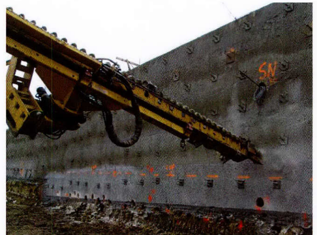
Figure 1. Soil Nail Wall.
