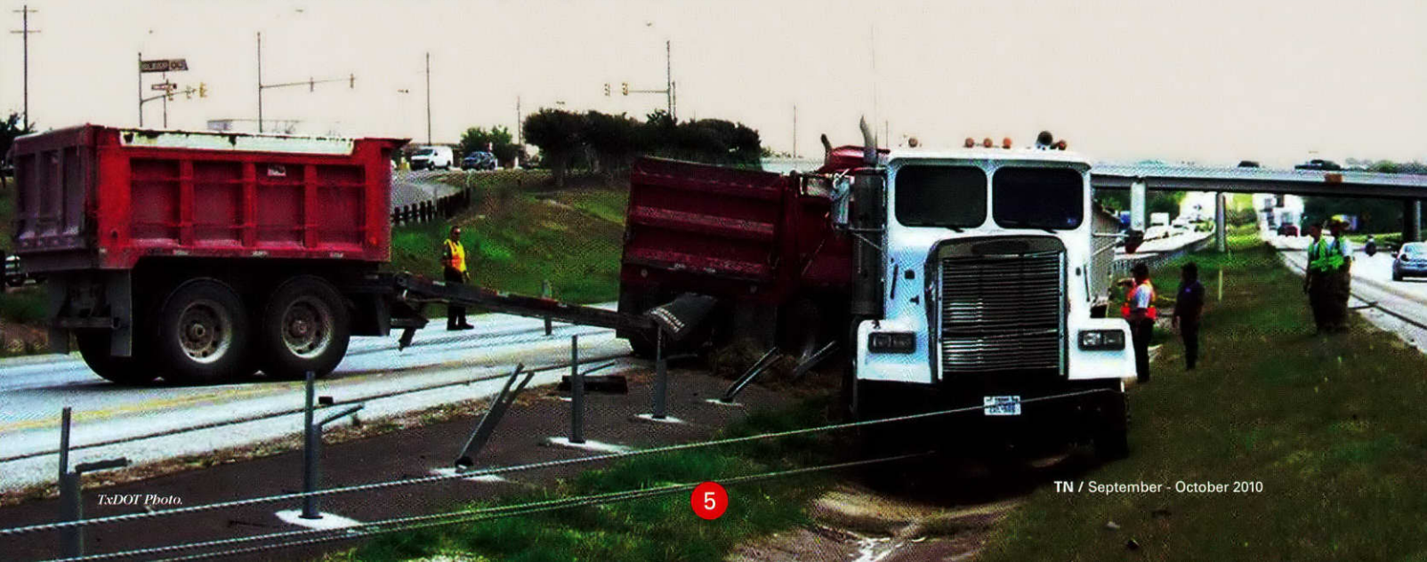
This stretch of I-20 in Parker County (Fort Worth District) was one of the first in the state to use cable barrier. Cable barrier systems are designed to stop passenger vehicles, but they are sometimes able to prevent large trucks from crossing the median.
