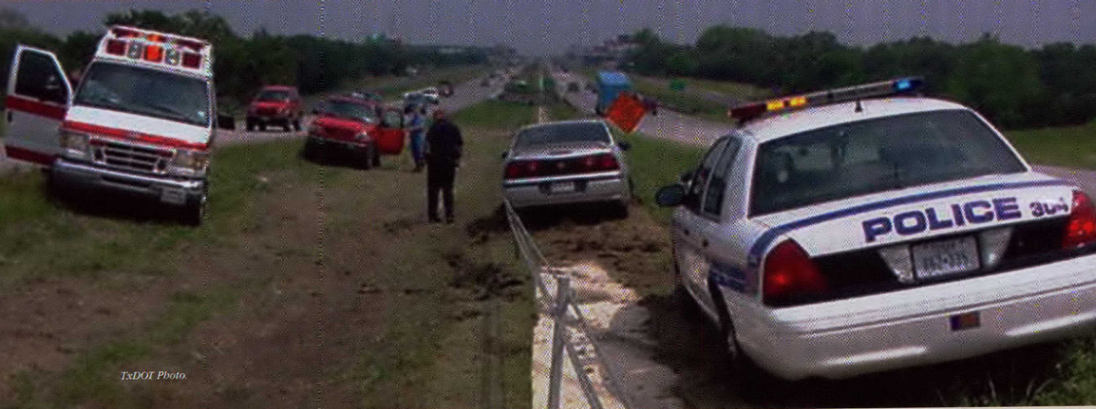
A driver is able to walk away after a cable barrier installed along I-10 in Kendall County keeps the car from entering the opposing lane of traffic.
