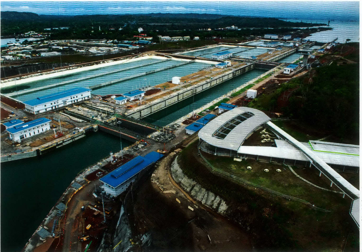
Water saving basins at the Agua Clara Locks, Atlantic side.
