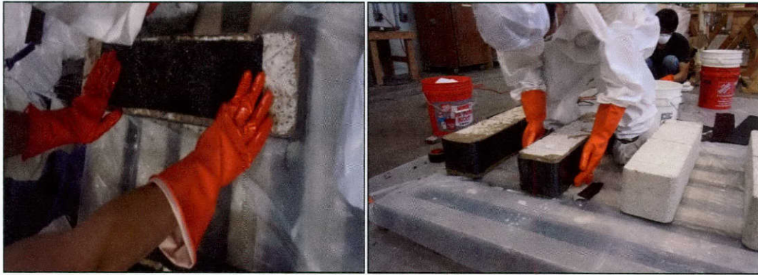
Figure 6-11: Applying CFRP strips
