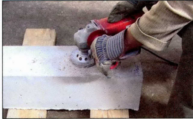
(a) Grinding a concrete surface
