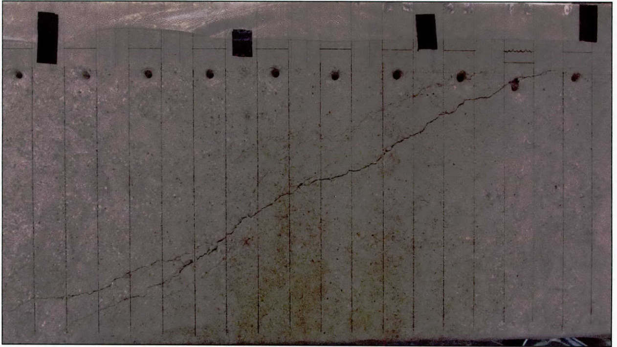
Figure 5-18: S-C-VA-HN crack pattern prior to CFRP installation
