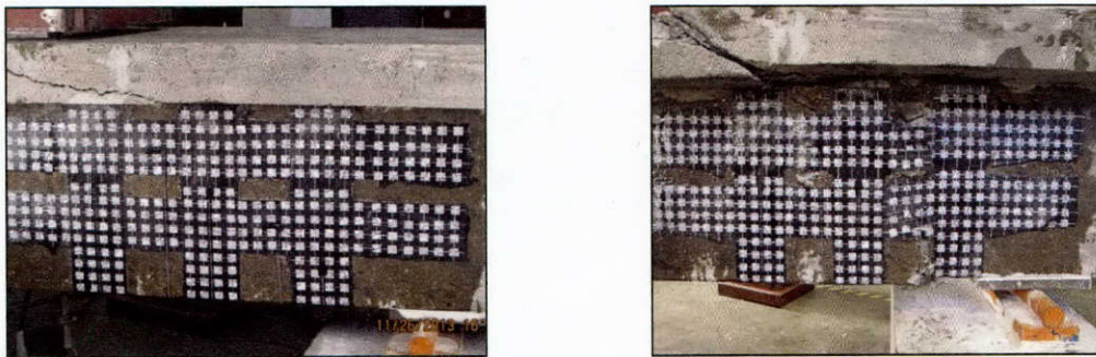
(b) Concrete Crushing Failure
