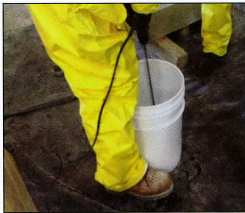
Figure 6-9: Mixing the epoxy components (Huaco, 2009)
