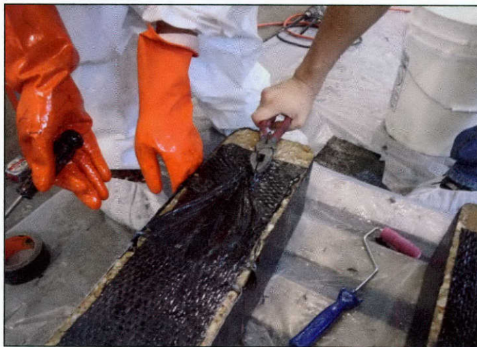
Figure 6-12: Fanning the anchor
