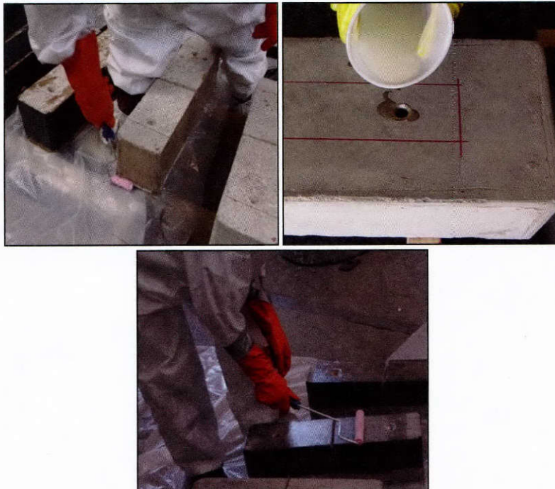
Figure 6-10: Saturating holes and surfaces (Hauco, 2010)
