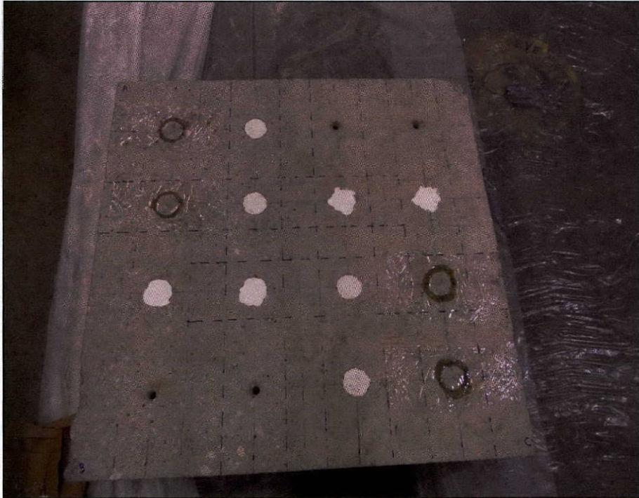
Figure 7-7: Concrete slab before installation of CFRP strips and anchors
