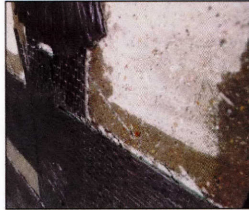
(e) Debonding horizontal strip
