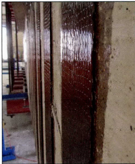
Figure 3-47: Debonding of strips in 48-3-14-3
