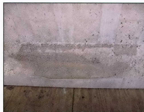
(b) After repair
