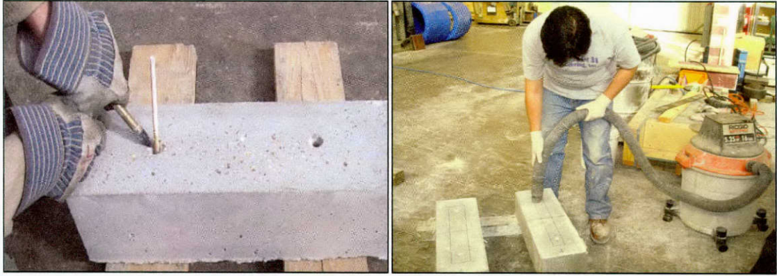
(d) Cleaning holes with compressed air or vacuum cleaner Figure 6-6: Specimen preparation before CFRP installation
